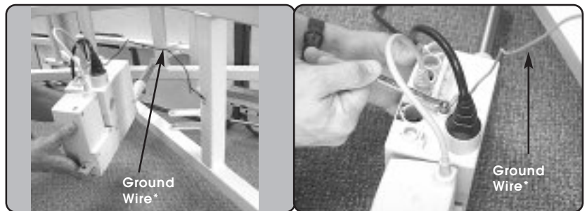
Removing Electrical Plugs and Ground Wire
